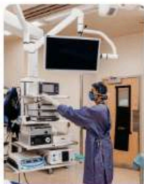
Operating Room Video Equipment
